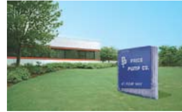
Price® Pump Co. manufacturing facility in Sonoma, CA.
